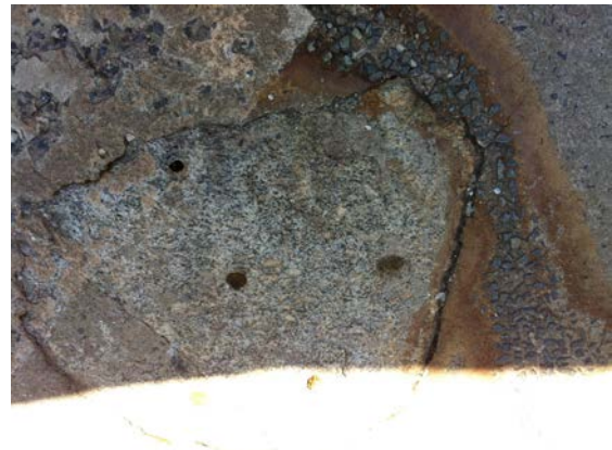
Image 12 Exposed aggregate at base of observatory (ACT Heritage 2015)
