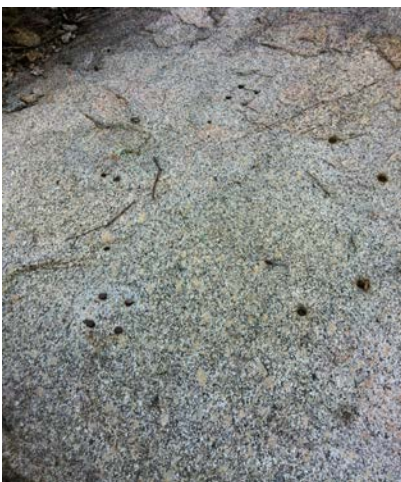
Image 4 Cut-off poles drilled into rock. Used to mount equipment (ACT Heritage 2015)
